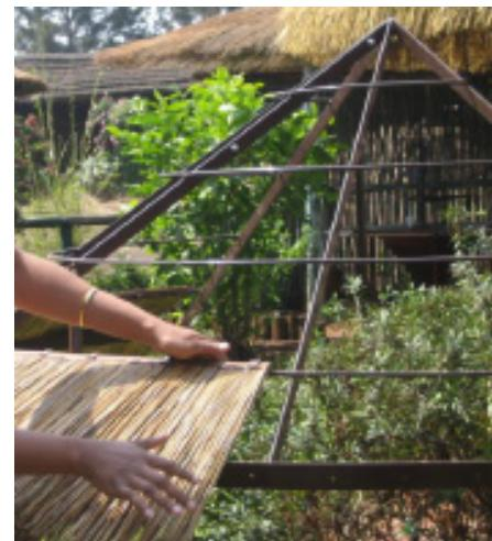
**Step 5:** Place the roof cone along the outer centre ridge of the frame, if necessary with the aid of a broomstick. For large models, you can first place the roof cone on the frame and raise it to affix the last reed panels. To keep the cone in place, attach it to the frame with the ties provided for this purpose.
